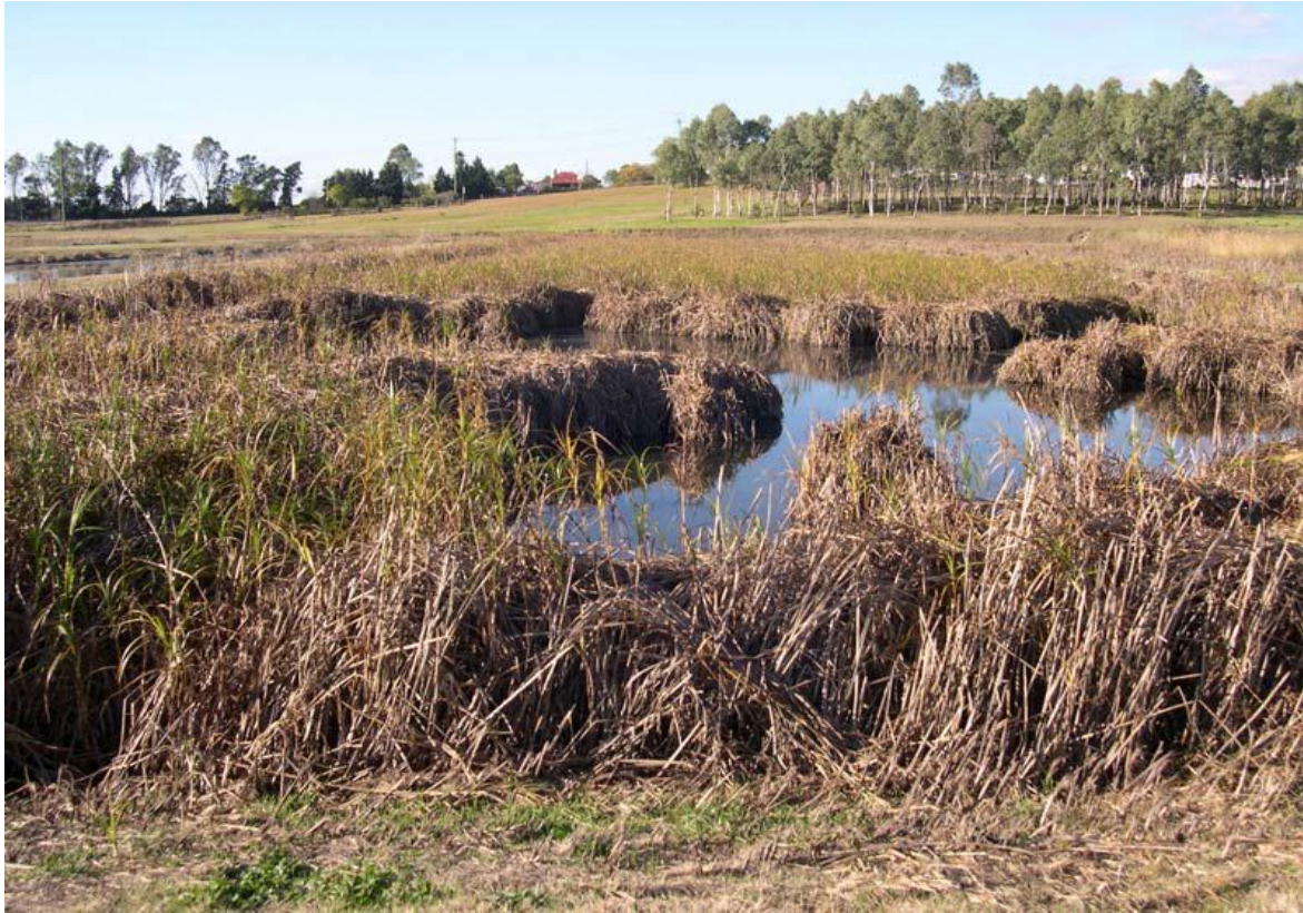
Figure B2.A FWS CW for tertiary treatment of municipal wastewater
